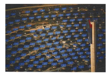
But contrary the CAT this project use sampling technique. The face of the wavefront comes thanks to the huge primary mirror in different times at individual heliostats and from these differences in arrival times we are able to reconstruct original wavefront and from its proportions is possible to determine energy and trajectory of initiated cosmic ray particle.
