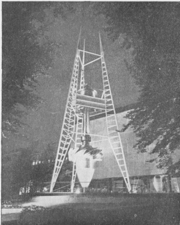
173. Suspension structure for Kaplan turbine.
