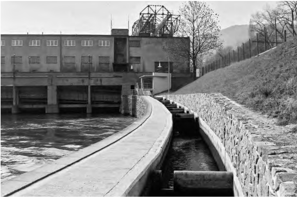
The new lowland pool fishpass at Střekov. (Photo by K. Halačka)
