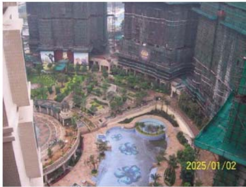
Picture 3: Buildings under construction
