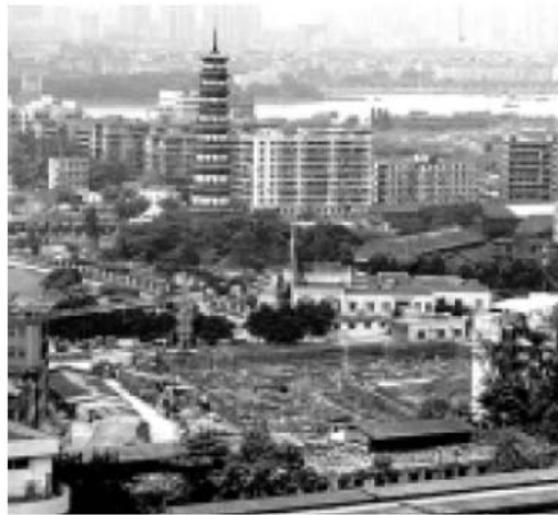
Picture 2: View before the site development
