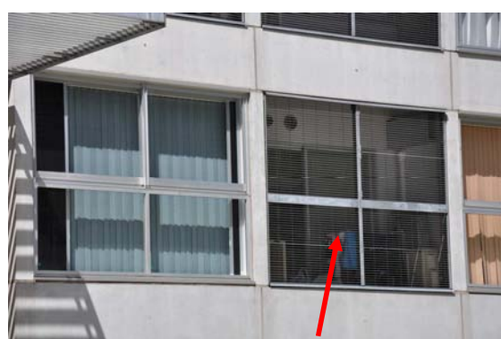
Private loggia behind metal latticework.
