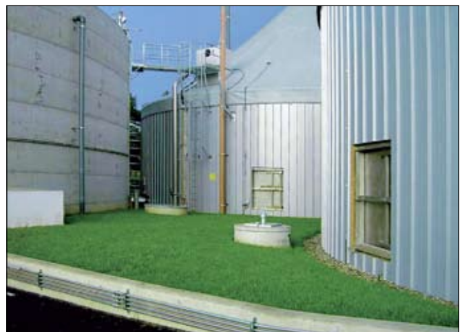
Biogas device (source: Renergy, s.r.o.)
