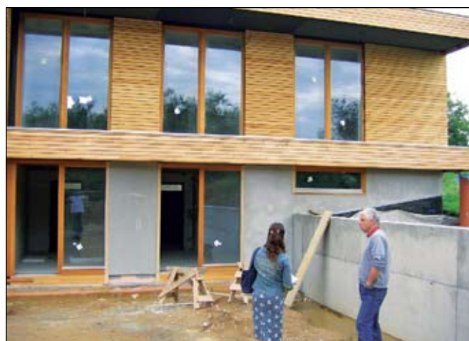
Prefabricated Wooden Panels House (source: Technology Centre ASCR)
