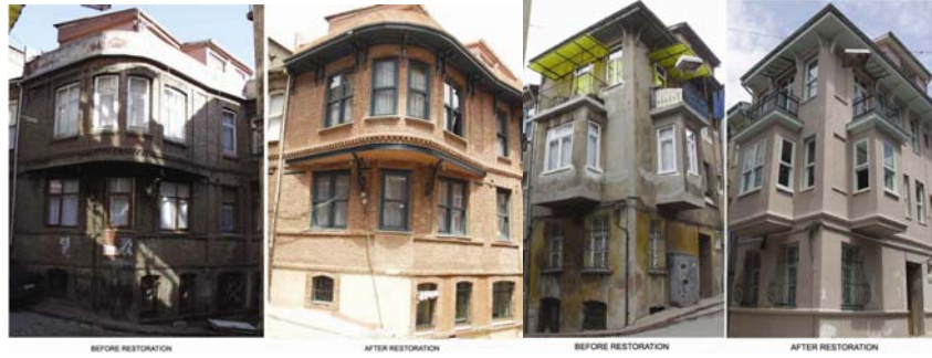
Figure 5. Restoration Samples from the Fener Balat Districts Rehabilitation Programme (Res: http://www.fenerbalat.org )
