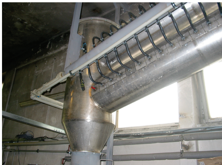
Wet separator for flying ash
