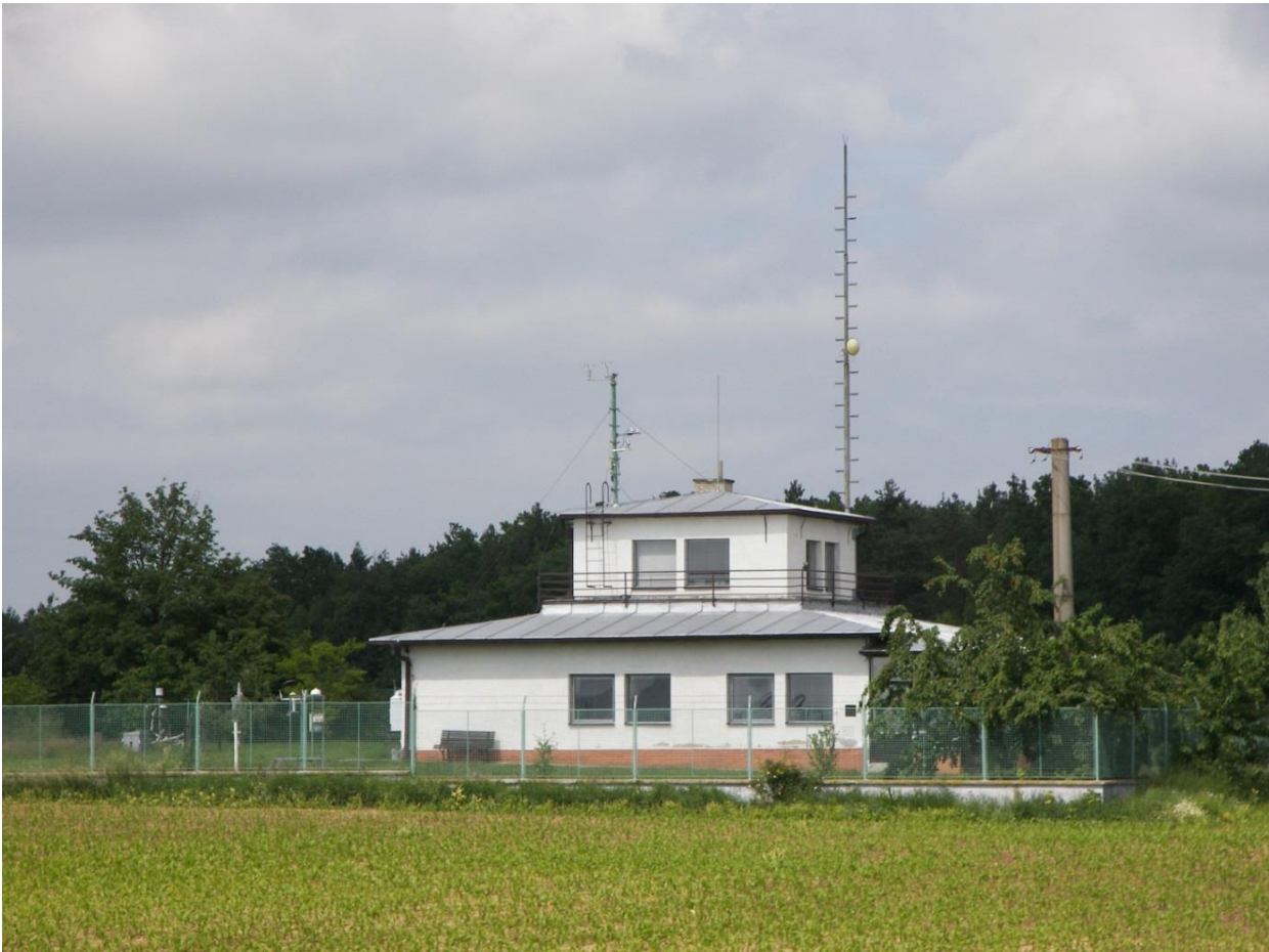
Figure 6 The typical manned weather station Kuchařovice. The observed wind climate is affected by the anemometer position above the rooftop, by the forest behind (its potentially strong effect is limited by low frequency of wind direction from the forest), by near-by trees, a wind mast and a parallel anemometer.
