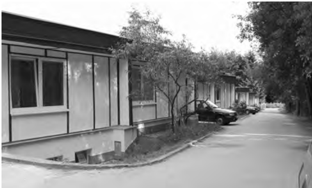
Dwelling bungalows at Studenec after reconstruction.
