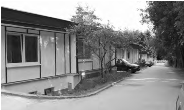
Dwelling bungalows at Studenec after reconstruction.
