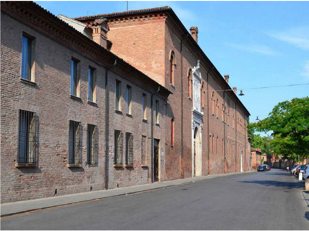
11. Palazzo Schifanoia, Ferrara, general view.
