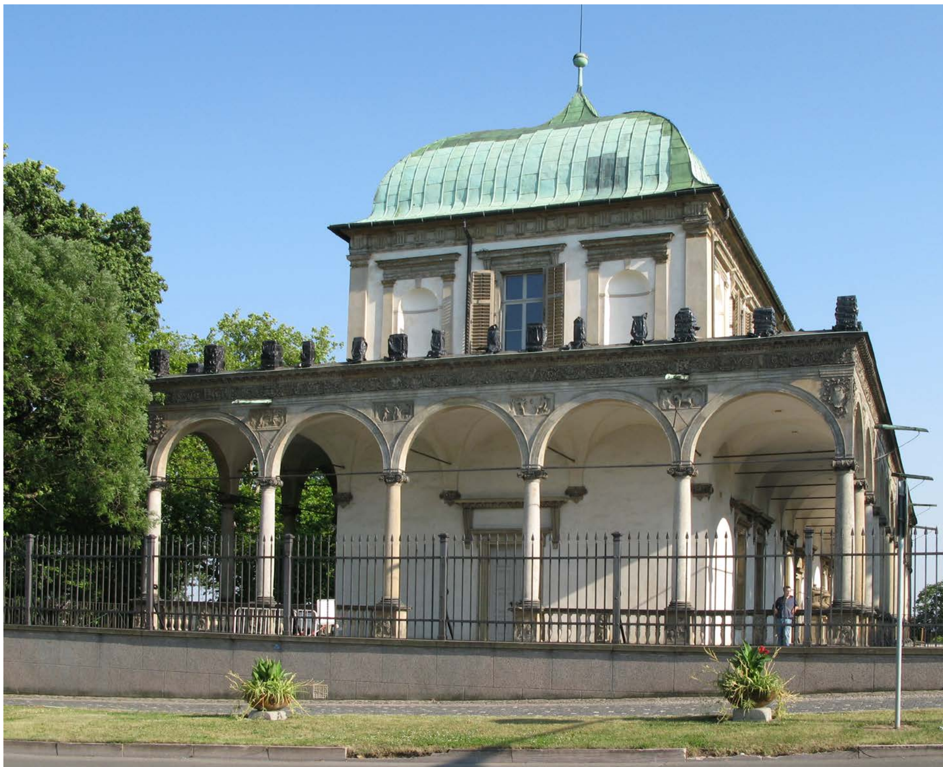
1. Belvedere, north facade during a reconstruction, without stone balustrade showing the arcades and windows and doors behind them.
