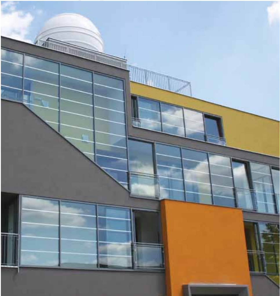
The headquarters of the Institute – Prague worksite.
