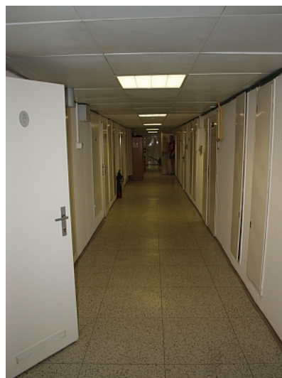
Stav chodby v 1. PP
