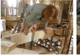
Fig. 29 Preparation of a groove for a key using a hand saw
