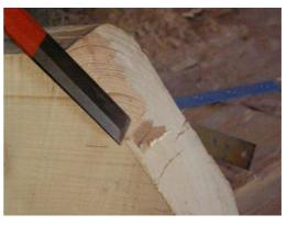
Fig. 32 Cutting off the excess length of the scarf joint
