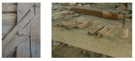
Fig. 37 Wooden nail in the joint (left), wooden nails removed from the joint (right)
