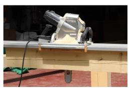
Fig. 22 Cutting a longitudinal scarf joint by a carpentry chainsaw
