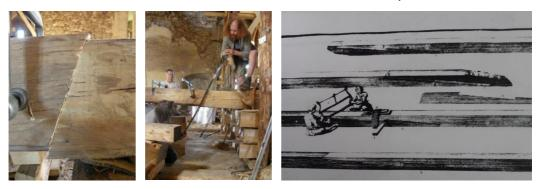
Fig. 33 a) Putting the joint faces together, b) cutting through by a handsaw c) cutting through the joint faces [19]
