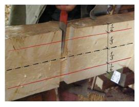
Fig. 31 Undercutting two-thirds of the inner central part of the joint, contact surfaces remain only along the edges of the joint
