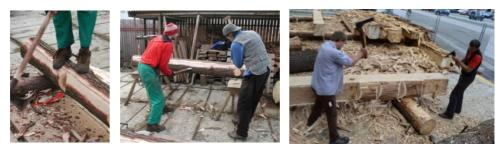
Fig. 41 Notching (left, centre) [16], rough hewing (right)
