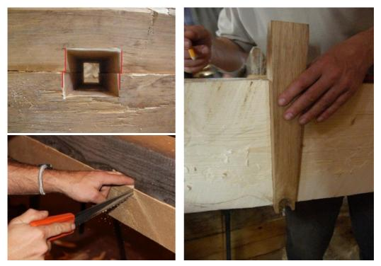
Fig. 34 a) Cutting grooves for keys with offset allowing shoring of faces when tightening keys (highlighted in colour, top left),
