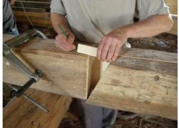
Fig. 30 Marking the oblique face according to already prepared counterpart
