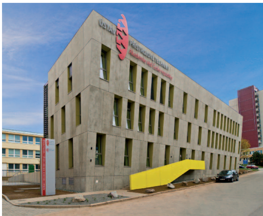
New infrastructure – ALISI, front view
