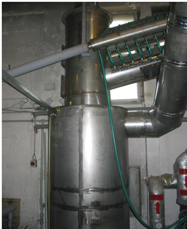
Wet separator for flying ash
