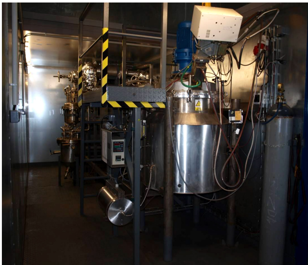
Pilot equipment for microwave thermal desorption (Dekonta a.s.)
