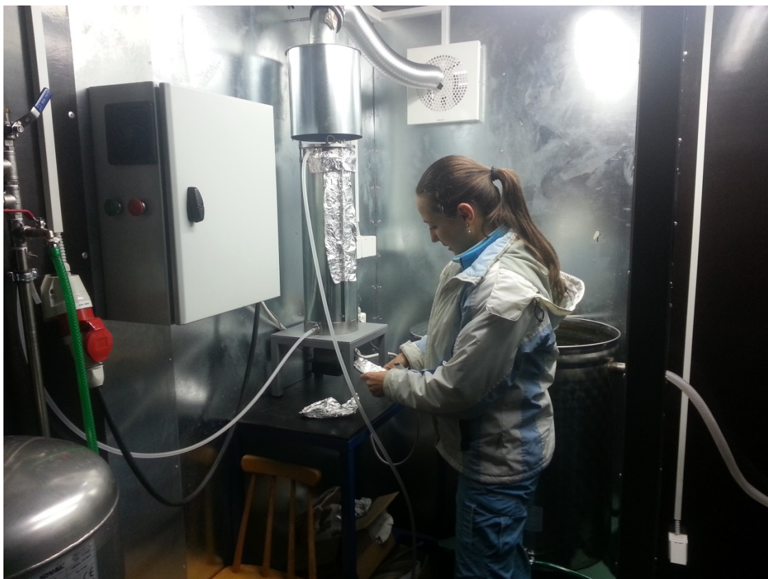
Operational tests on sewage plant
