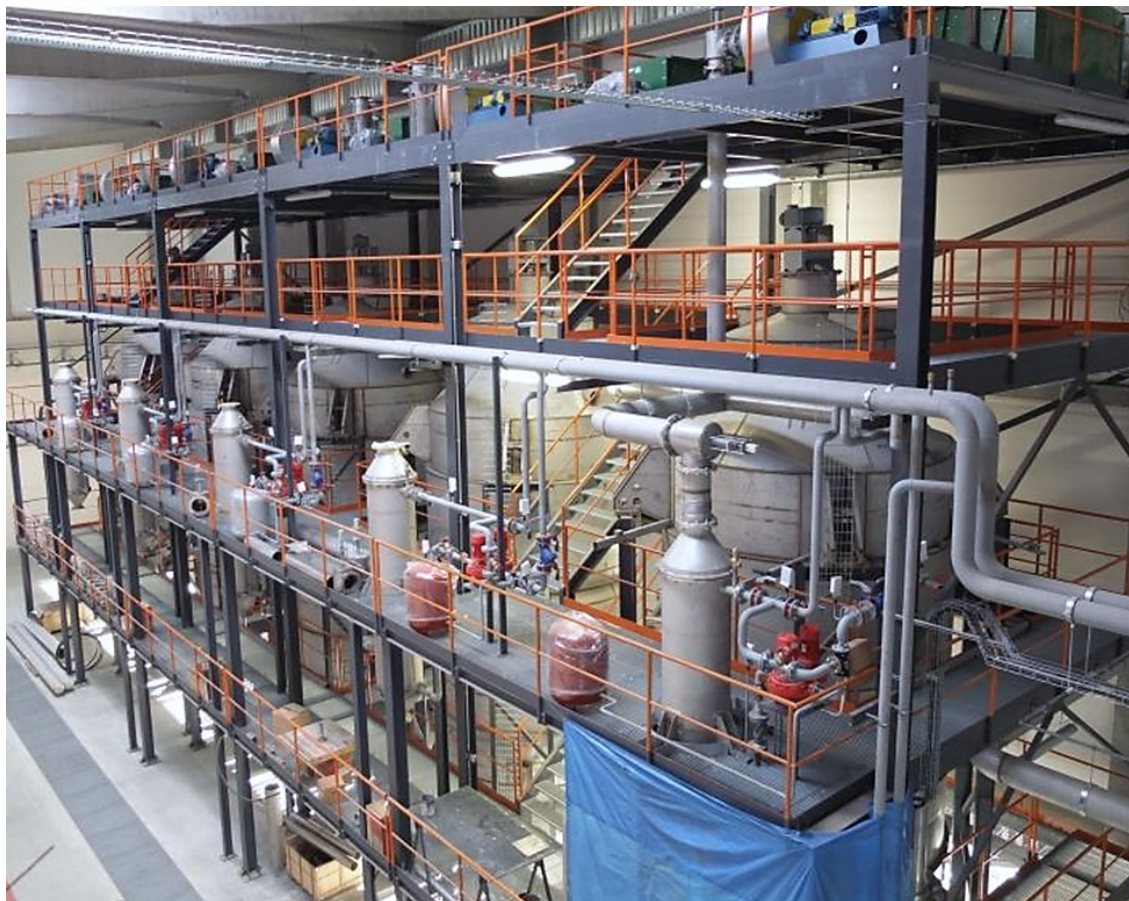
Combined heat and power generation plant in Kozumín – under construction
