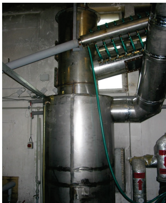
Wet separator for flying ash
