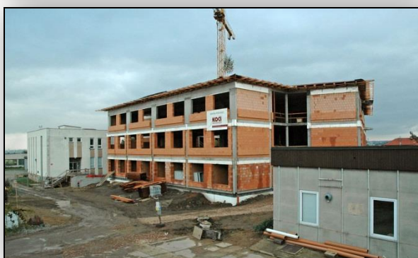
Construction of a new building.
