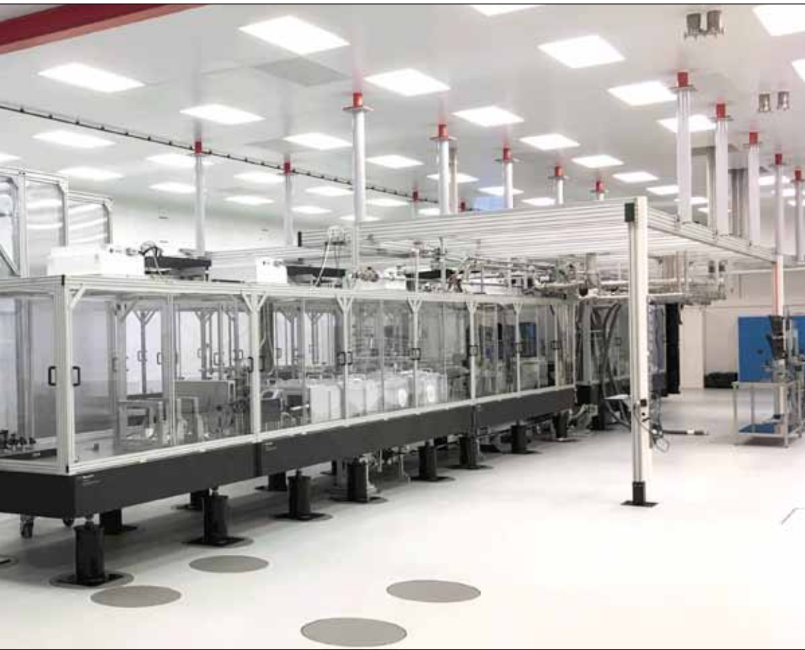
The L3 laser system during installation and activation
