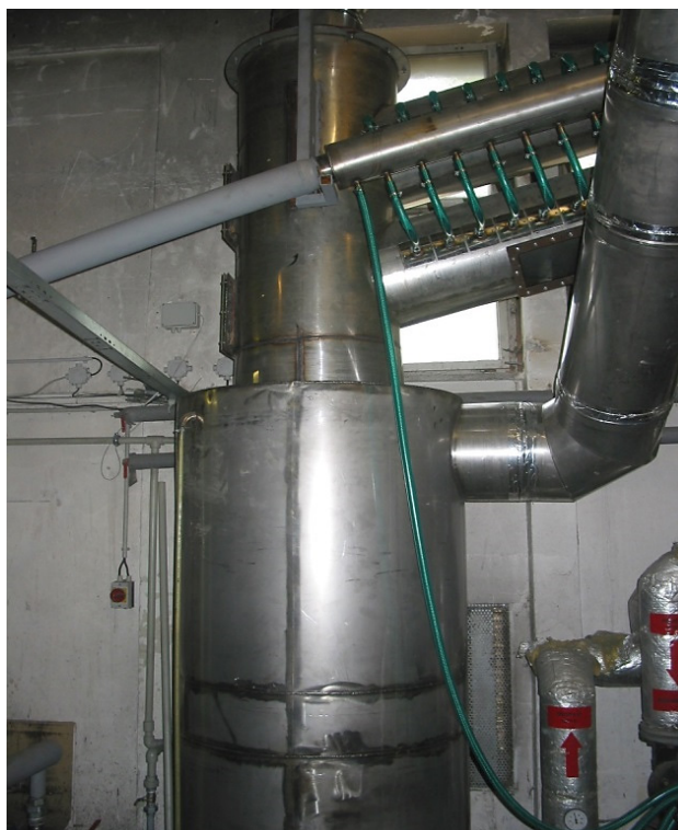
Wet separator for flying ash
