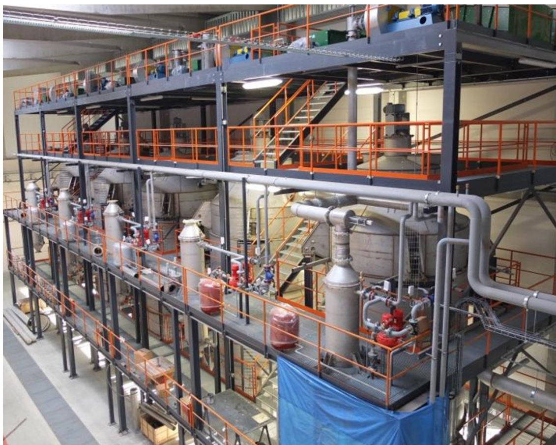
Combined heat and power generation plant in Kozumín – under construction
