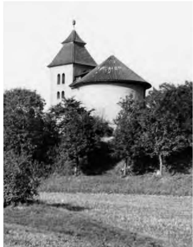
▲ Fig. 3. Budeč, Sts Peter and Paul Rotunda (from SW). The round nave of the church represents the earliest preserved building (from the foundations up to the vault) on our territory, the St Peter Rotunda, founded by Duke Spytihněv I (894/5–915) of the House of Přemysl.
