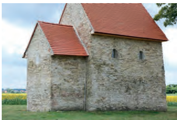
▲ Fig. 1. Kopčany – Chapel of St. Margaret of Antioch. From the north-east, condition after removing plastering in 2008. Photo by L. Poláček.
