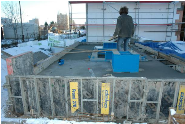
Fig. 3.5: Finished flywheel generators basement.
