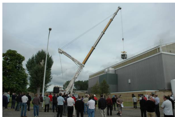
Fig. 1.3: The COMPASS-D tokamak lifting (outside view on crane).
