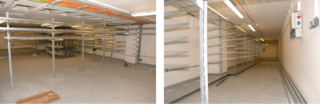
Fig. 3.12: Heavy current cabelling is under work.
