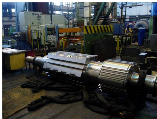
Fig. 3.2: Rotor of the generator is assembled in CKD Nove Energo
