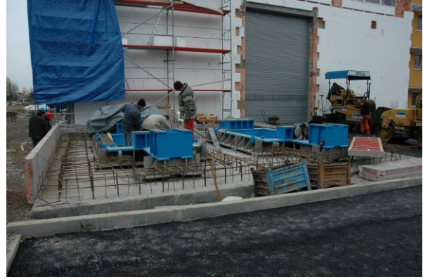
Fig. 3.4: Two special frames for the flywheel generators are installed
