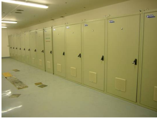
Fig. 3.8: Convertors for toroidal and poloidal circuits including their control.
