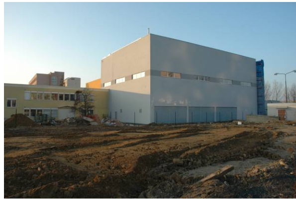
Fig 2.2: Tokamak building - north view.
