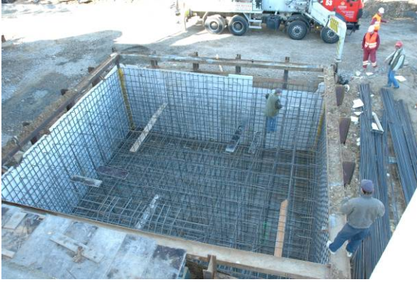
Fig. 3.3: Basement (re-inforcement) of flywheel generator
