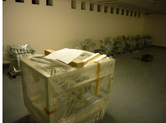
Fig. 3.9: Tokamak basement – deprecated chokes (back) and the crowbar system (front).
