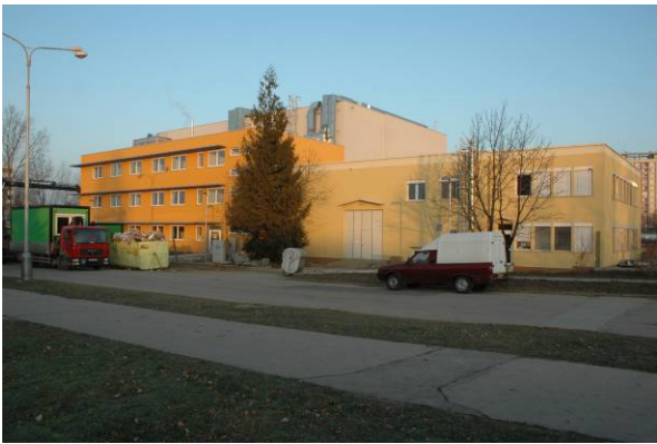
Fig 2.1: Tokamak building - south view.
