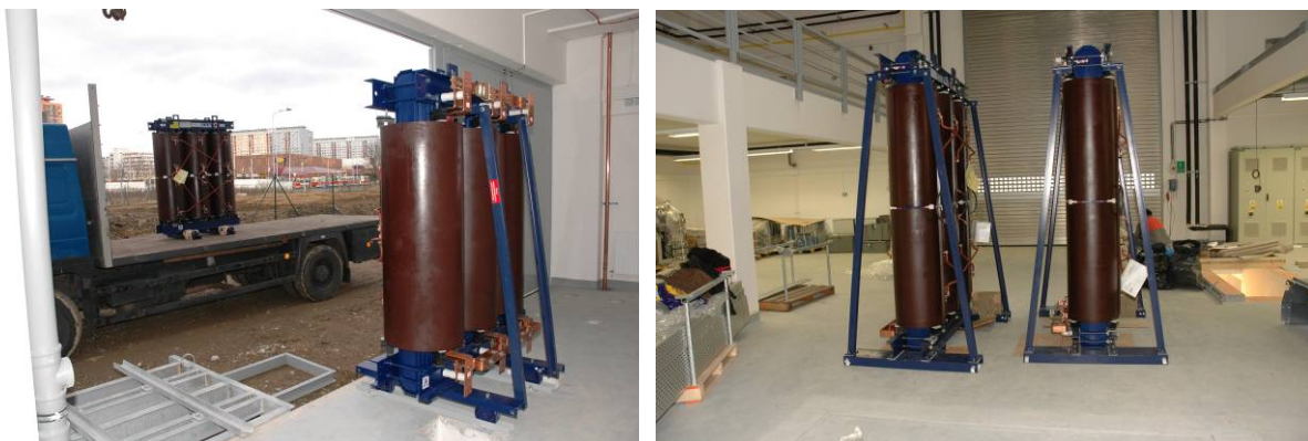
Fig. 3.11: Transformers have been delivered and are being installed.
