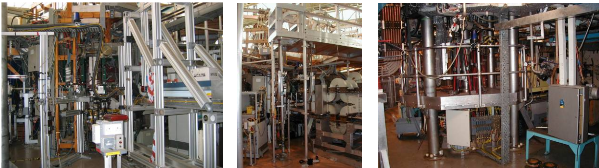
Fig. 1.1: COMPASS hall before start of dismantling
