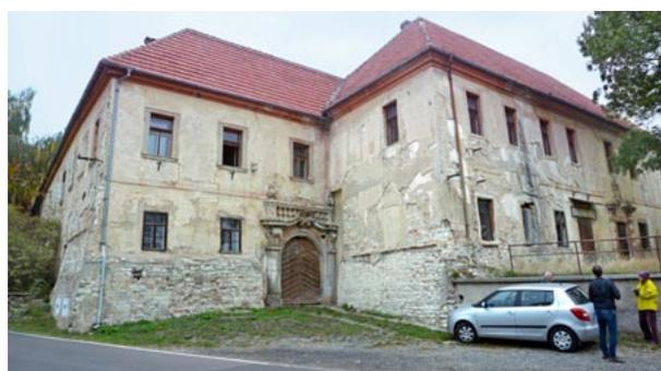
■ **Fig. 28.** The chateau at Zahořany, now in the need of reconstruction, results from three construction phases ranging from Renaissance period (southern wing, on the right) to modern times. Sandstone was used mainly for portals and for window sills. Photo by J. Adamovič.
