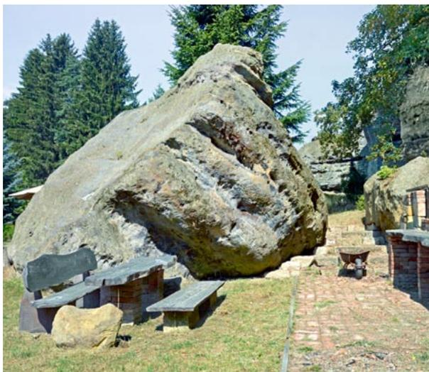
■ **Fig. 31.** This 150 m<sup>3</sup> rockfall at Juliovka from 2009 heavily damaged the previous house “U Galejníka”, which had to be demolished. The event was caused, among other factors, by artificial undercutting of the cliff face. Photo by J. Adamovič.
