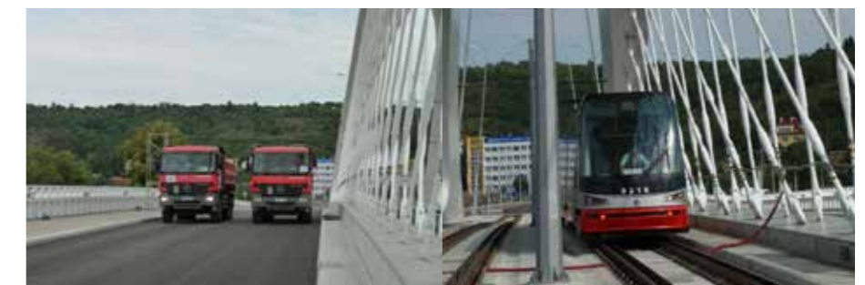
Basic dynamic load test is usually carried out prior to commissioning the bridge. It aims at the determination of the initial dynamic stiffness of the structure and vibration amplitude upon passage of testing vehicles. The picture shows an example of measurement on the Troja Bridge
