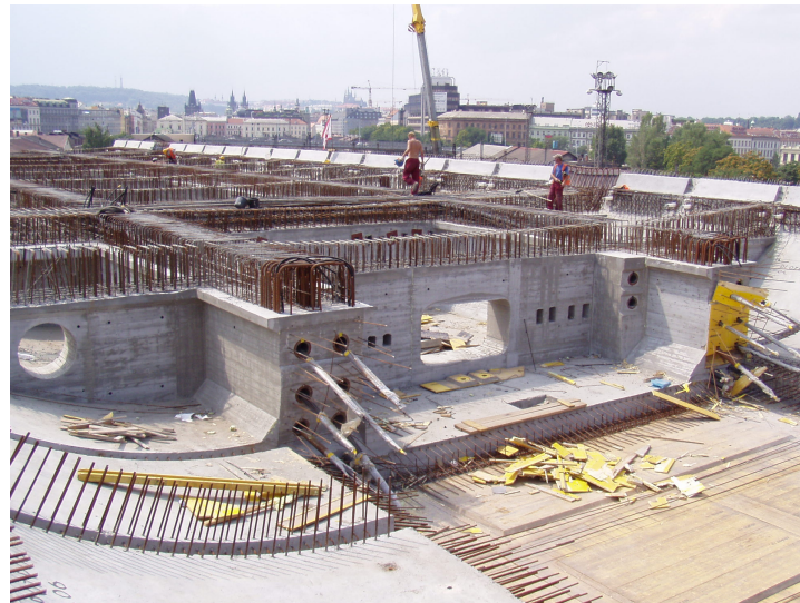
Figure 16: Construction of the scaffold bridge in Prague, photo by D. Prause.
