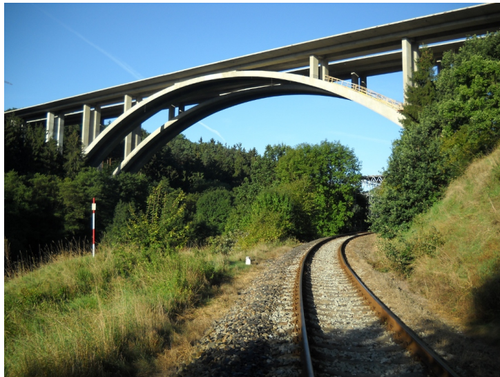
Figure 21: The Oparno bridge, Czech Republic, 2010.
