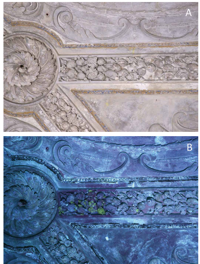
Figure 3: A view of the part section with glued transfers and accessories in daylight (A) and in UV light (B). Zinc whiteoxide, which was mixed in to the new supplements additions, fluoresces green.
