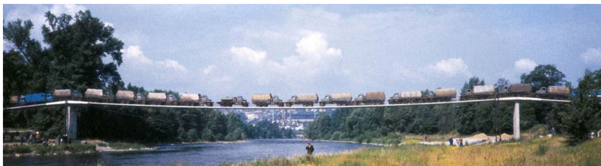
Fig.4.7.1 Prague-Troja Bridge - load test
