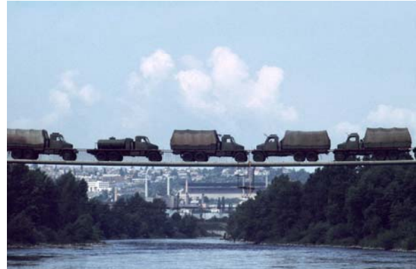
Fig.2.3 – Prague-Troja Bridge - Loading test
