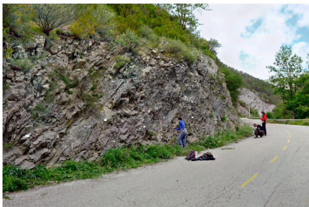
■ Fig. 7. The Compte I section near Baro in the Spanish Central Pyrenees with the Lochkovian-Pragian boundary. Photo by Leona Chadimová.
