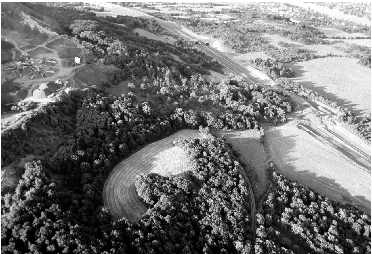
Fig. 1: Aerial picture of the mutual position of the quarry Dobkovičky and landslide.
