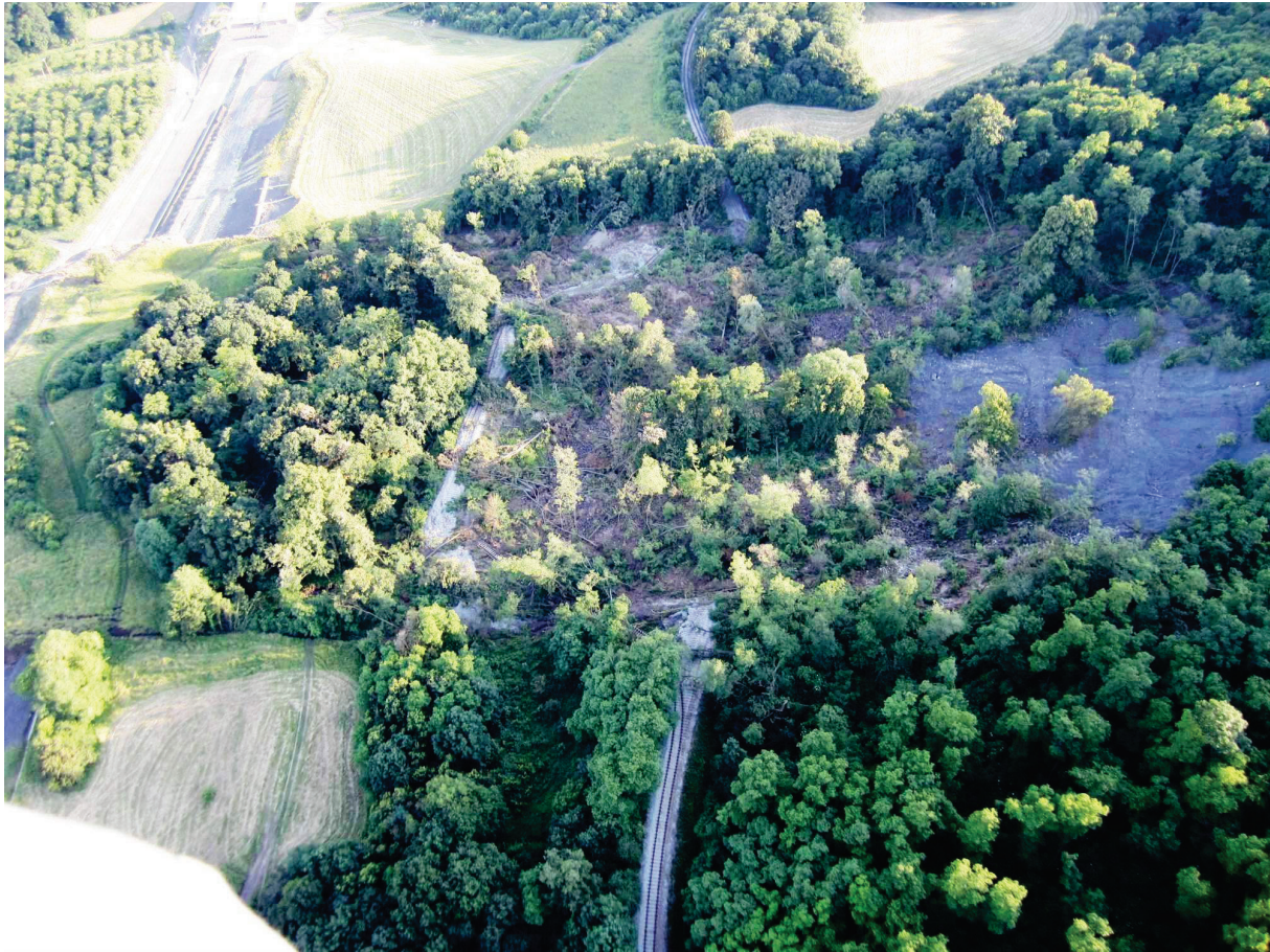
Fig. 2: The landslide area, smashed railway and buried motorway
