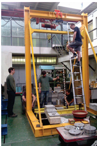
Fig. 1: Steel frame with hoist.
