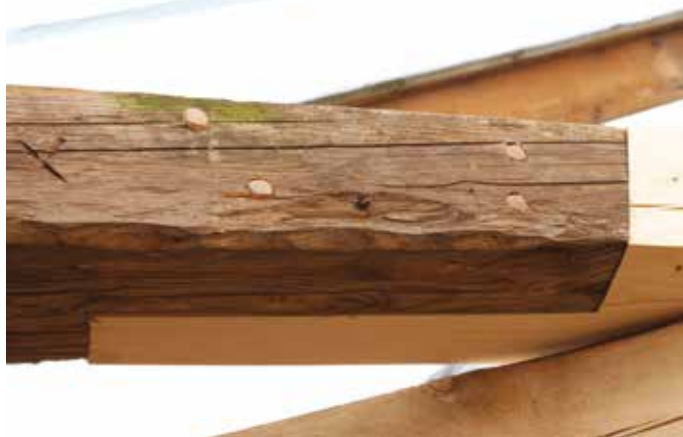
Use of all-wooden joint during reconstruction of rafters in Bratronice castle
