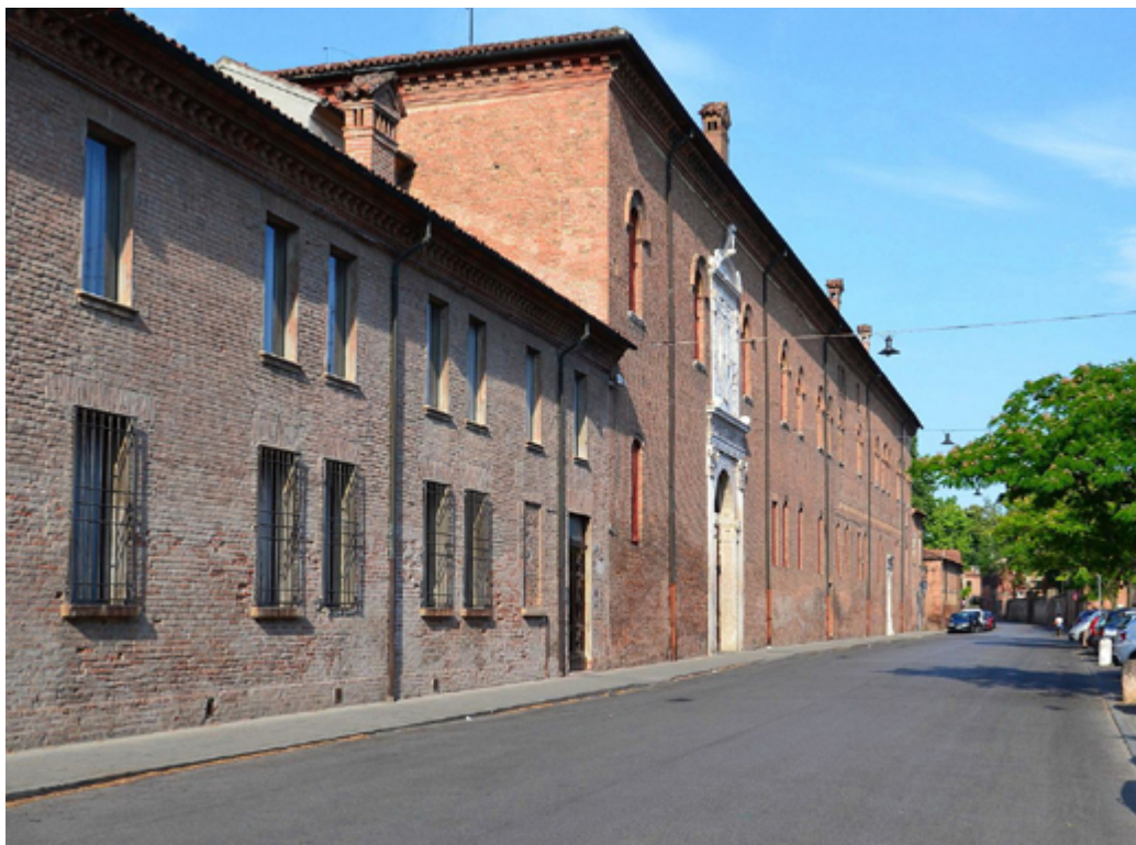
11. Palazzo Schifanoia, Ferrara, general view.
