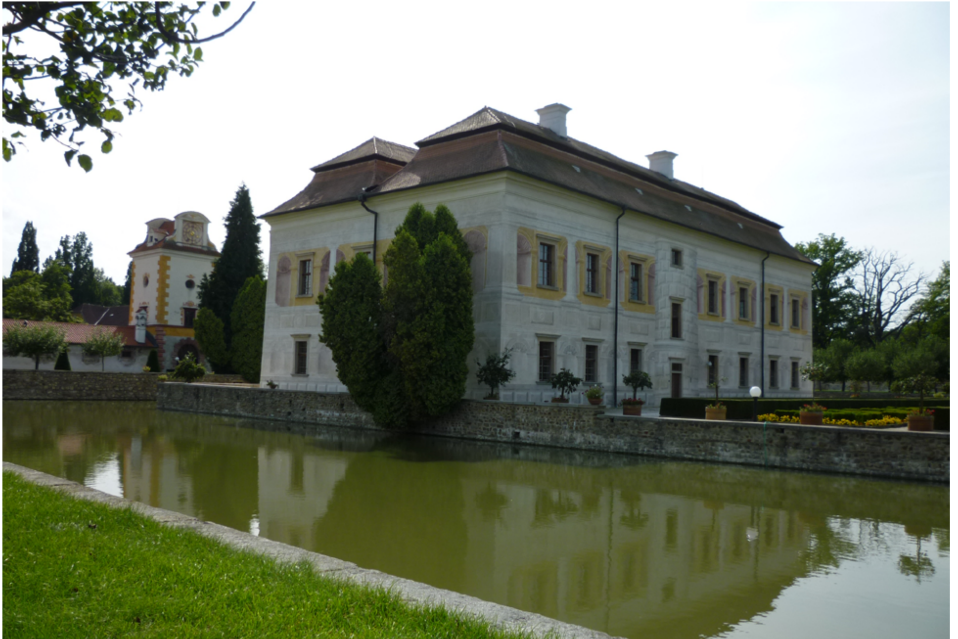
4. Kratochvíle villa. View of the central villa with the entrance tower, 1583–1589.
