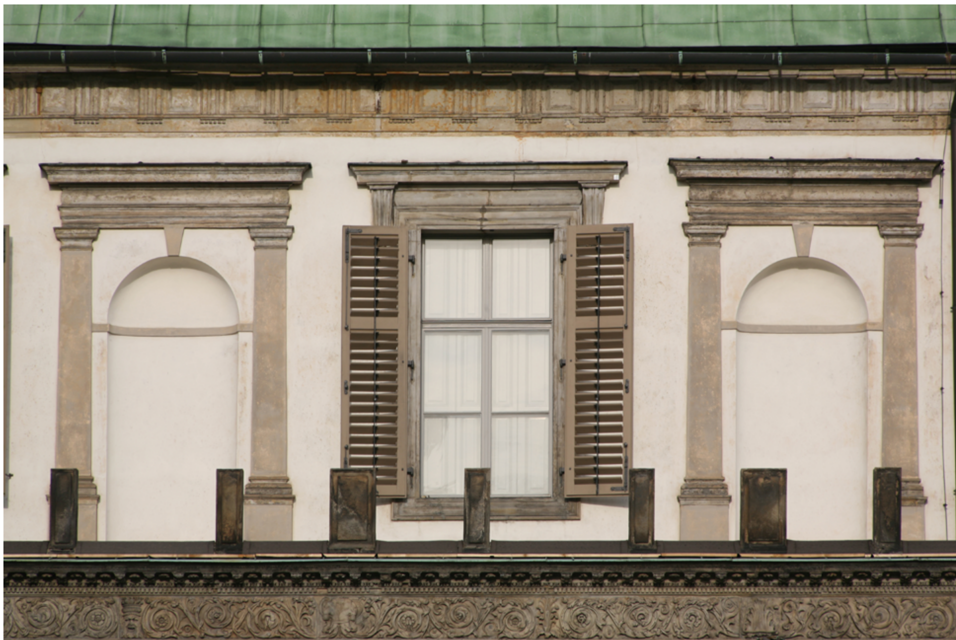
4. Photograph of the upper facade of the Belvedere, showing niche and window.
