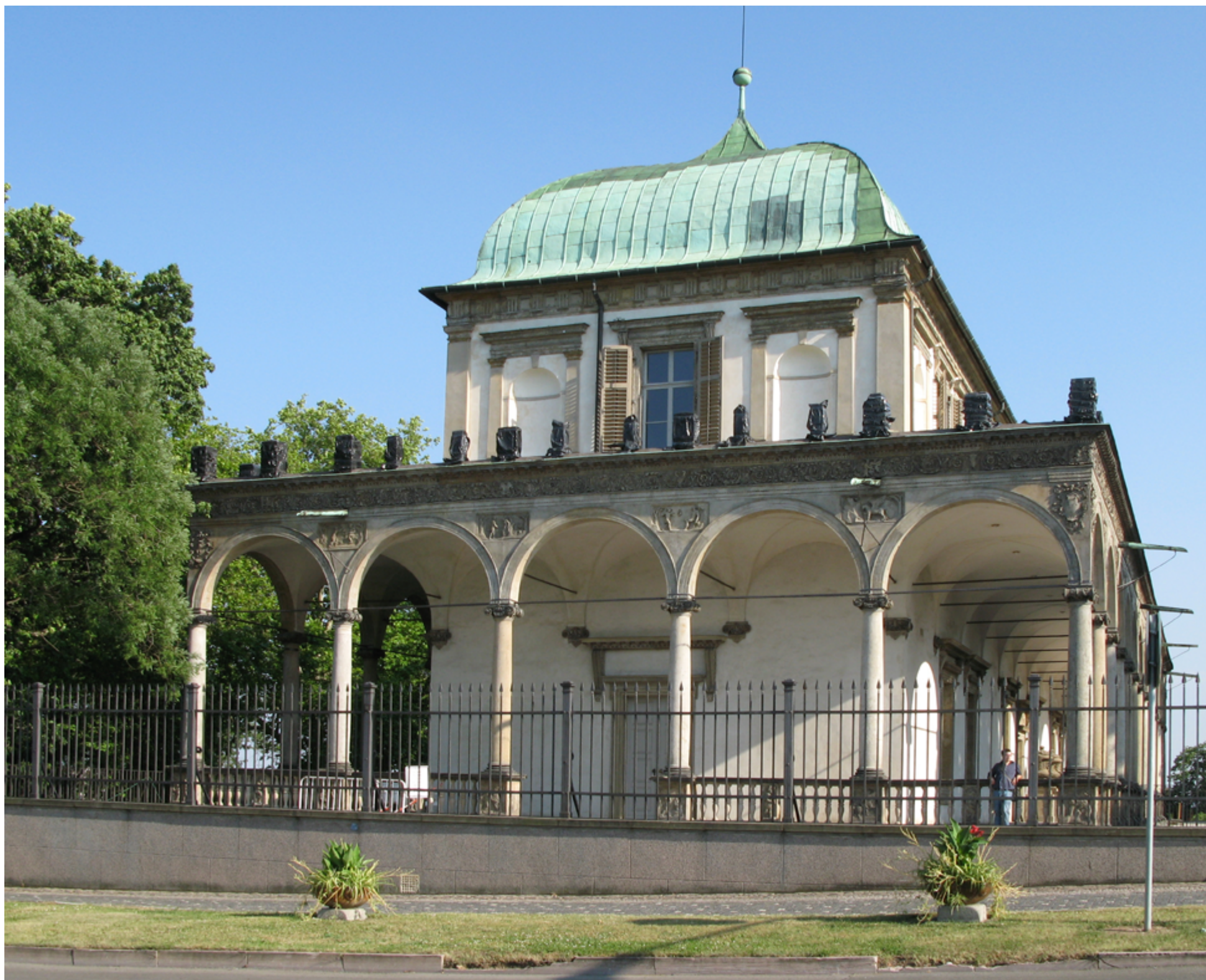
1. Belvedere, north facade during a reconstruction, without stone balustrade showing the arcades and windows and doors behind them.
