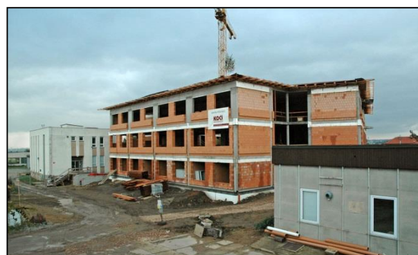
Construction of a new building.
