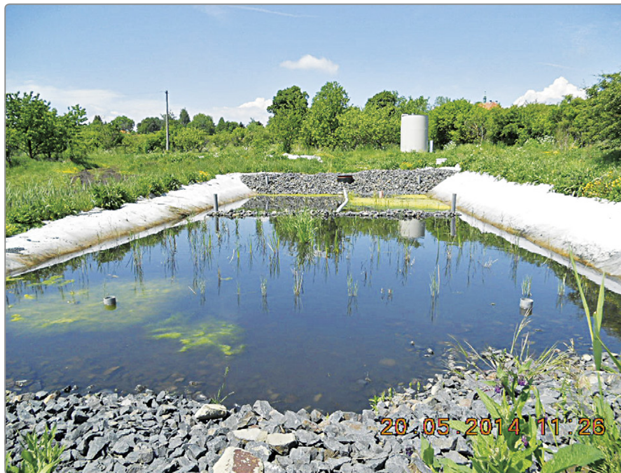
Figure 4: Accumulation and/or degradation of Praziquantel (PZQ) in plants were determined using Phragmites australis in vitro cultivated plants. In case of initial PZQ concentration 20 \text{ mg L}^{-1} , 90 % was removed from liquid media within 21 days. Laboratory results were confirmed in real scale using the constructed wetland (CW), where PZQ was completely removed until the first purification pond. This result offers a promising possibility to use CW for PZQ removal from agricultural as well as domestic waste-waters.
