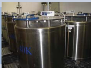
Liquid nitrogen storage vessels
