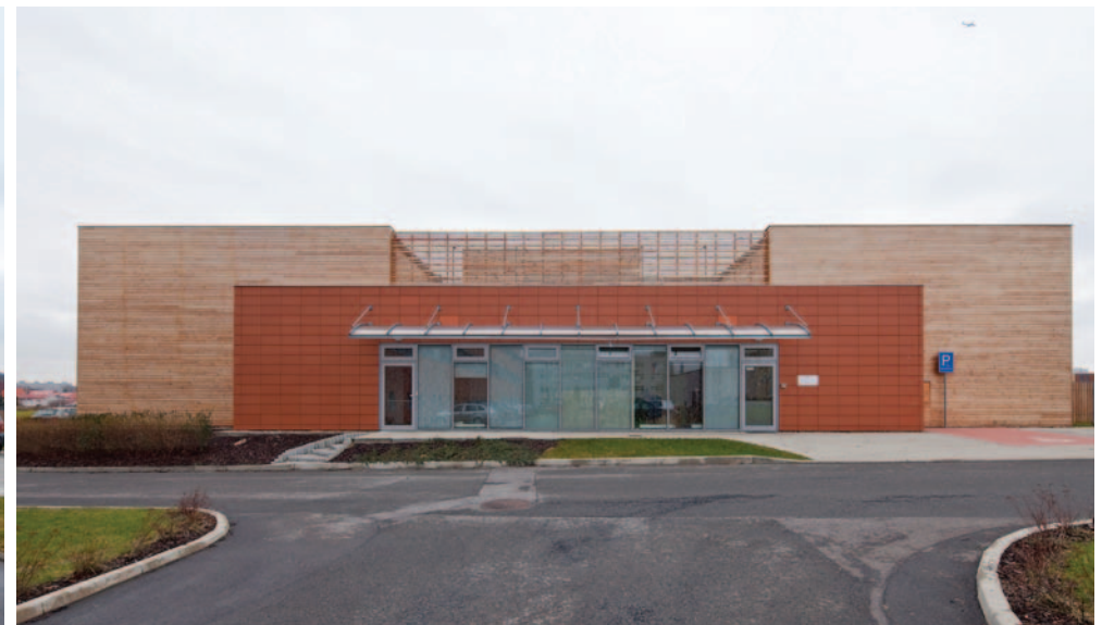
Entrance to the sports facility (left) and kindergarten (right)
