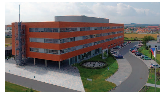
New building of the Institute in Prague 4 - Krč
