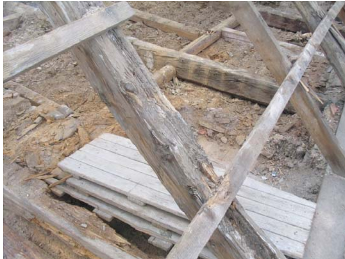
Fig. 1: View of the roof beam structure.
