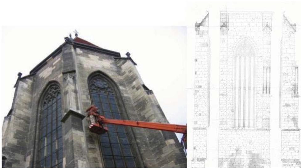
Fig. 1: Left - mapping and identification of individual building blocks, right - an example of existing paper facade plan (Vician et al., 1957).
