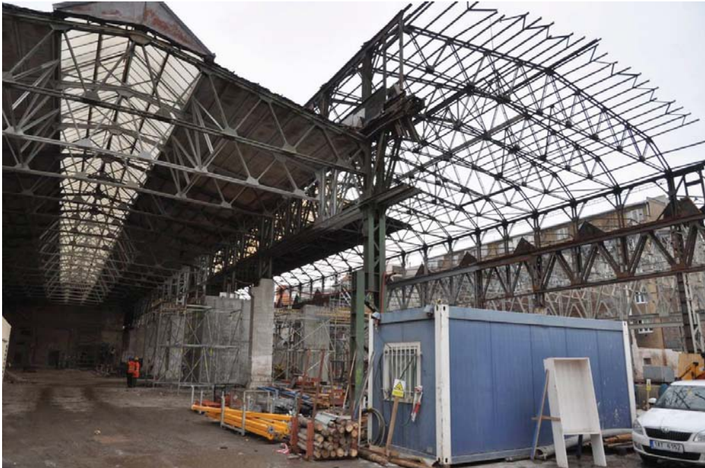
Fig. 1: Former factory for boiler production in Prague – Karlín under reconversion
