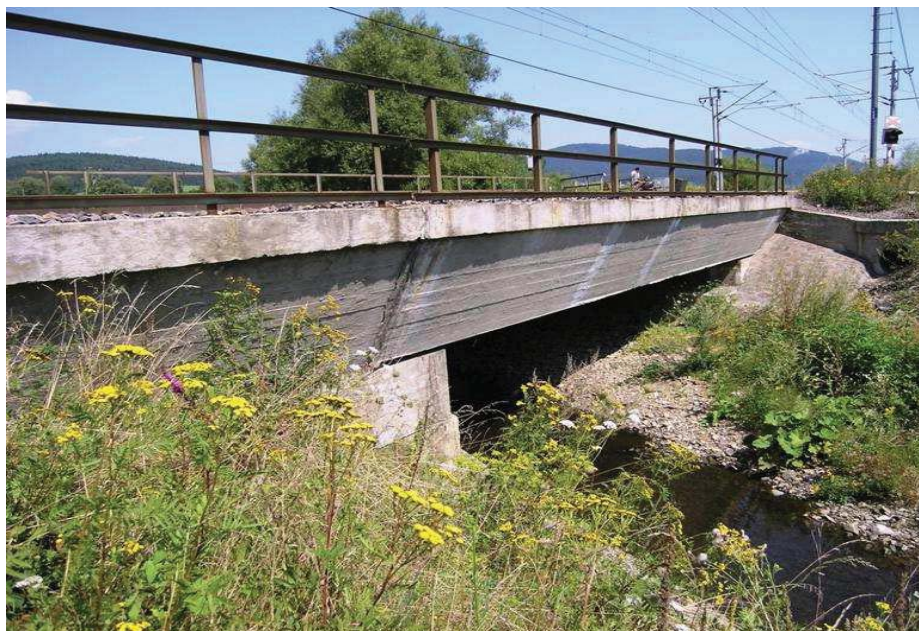
Fig. 1: View of the short-span bridge on ŽSR line Žilina – Čadca
