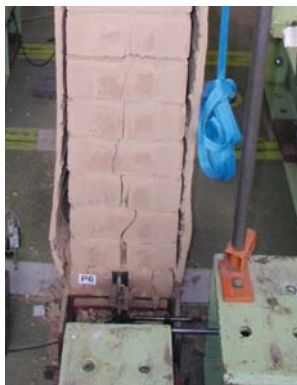
Fig. 15: Vertical crack in the wall thickness
