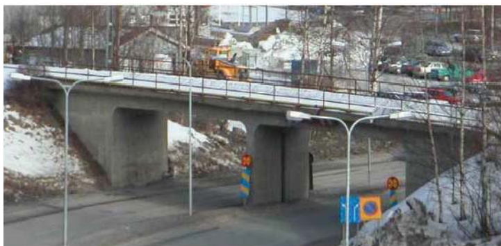
Fig. 1: Örnsköldsvik Bridge (Elfgren et al., 2007)
