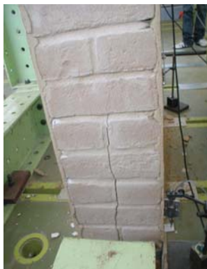
Fig. 13: Vertical crack in the wall thickness
