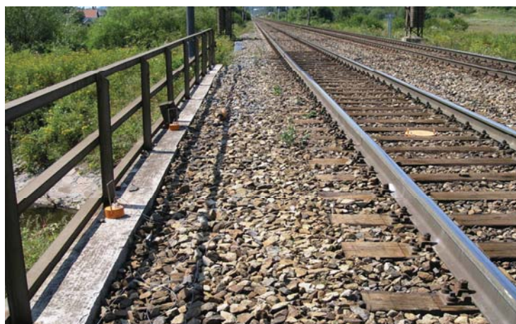
Fig. 7: Accelerometers with amplifiers – a part of CBMS
