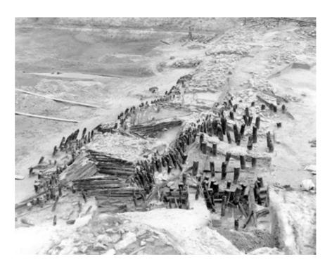
Fig.  $44\,$  A barrier at the bottom of the riverbed: a line of wooden caissons filled with stones (Channel 2).
