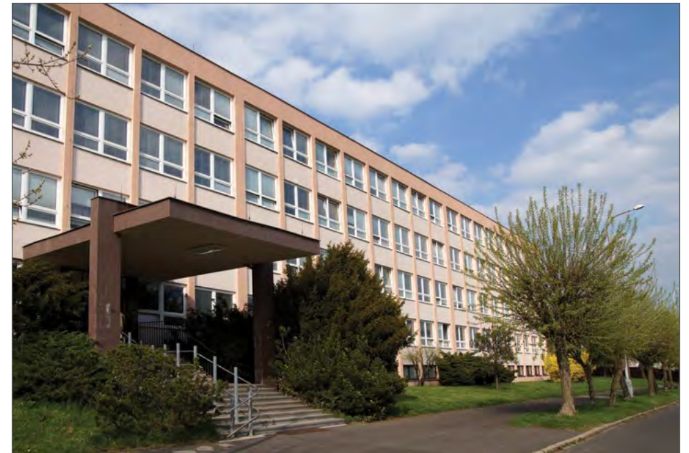
Fig. 2: The building in the street Na Slovance was built for the needs of the growing Institute of Physics which moved there in 1970
