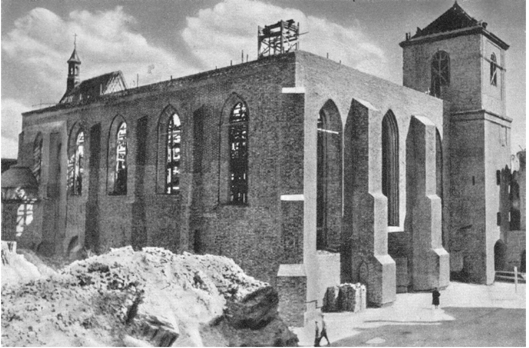
⬆ Fig. 11. Warsaw Cathedral during reconstruction, around 1950 (photo Alfred Funkiewicz, public domain)
