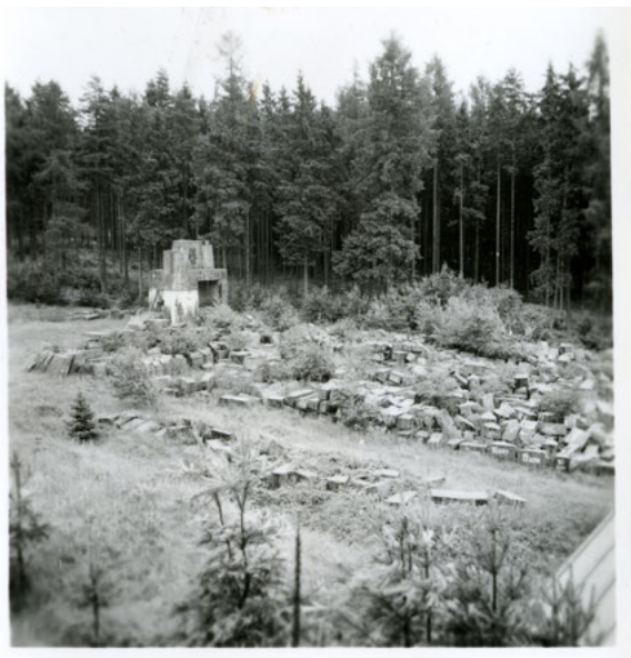
◀ Fig. 6. Podolsko u Písku, temporary location of the numbered parts of the bridge above the border of the floodplain, 1964 (Photoarchive of the National Heritage Institute, Regional Office in České Budějovice)
