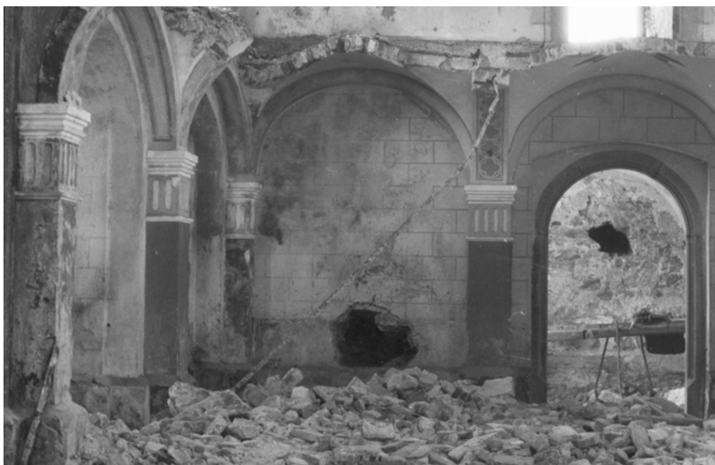
⬇ Fig. 6. Church in Kapličky before demolition, 1959 (Security Services Archive, Collection of photoalbums and photographs)
