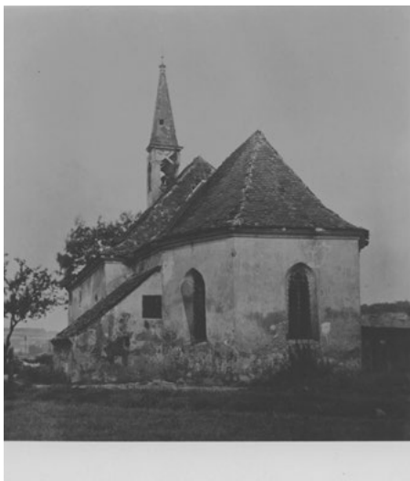
⬅ Fig. 2. View of the damaged church of St. Jošt in Cheb (photoarchive of National Heritage Institute, Directorate-General, Nr. N090456)
