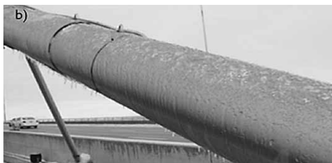
Fig. 1. Examples of icing and rope damage from aeroelastic oscillation.
