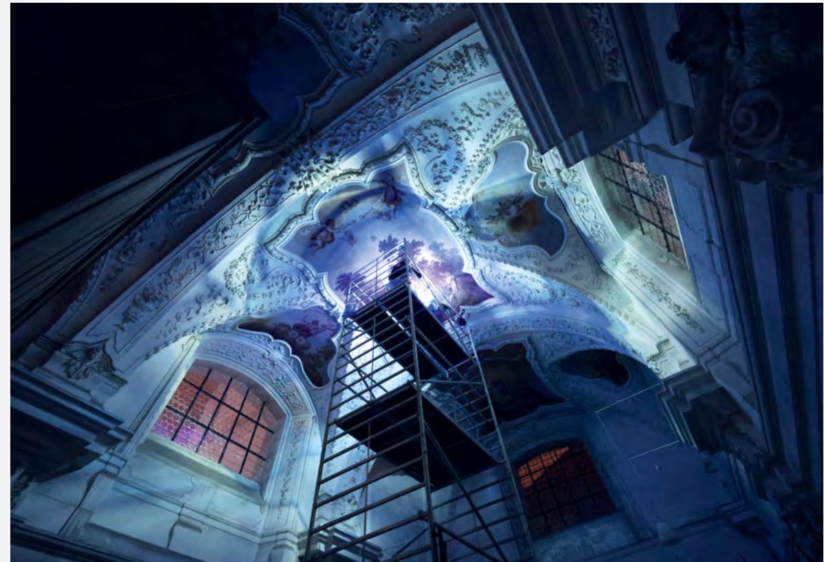
Survey of the baroque ceiling paintings by Johann Hiebl in the Doksany monastery church.
