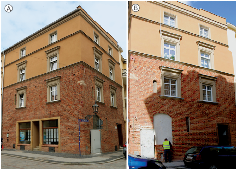
Fig. 74. Brzeg, 6 Jabłkowa Street. Corner townhouse from the 13th century (Vendic way house). A – After conservation works; B – at the time of conservation works. Photo by M. Chorowska.
