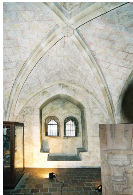
Fig. 108. Brno, 8 Radnická Street (Old Town Hall). Vaulted first-floor chamber with a segment of keystone. Photo by D. Merta.
