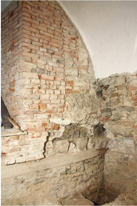
Fig. 127. Jihlava, 16 Masarykovo Square. A view of the south wall of the house with preserved cellar ceiling beams from 1259/1260. Photo by Archaia Brno, Inv. No. 352-2012.
