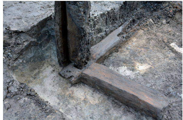
Fig. 49. Wrocław, 6 St Wita Street. Construction details of the northeast corner of a timber frame building. S. u. 247. Photo by P. Duma.
