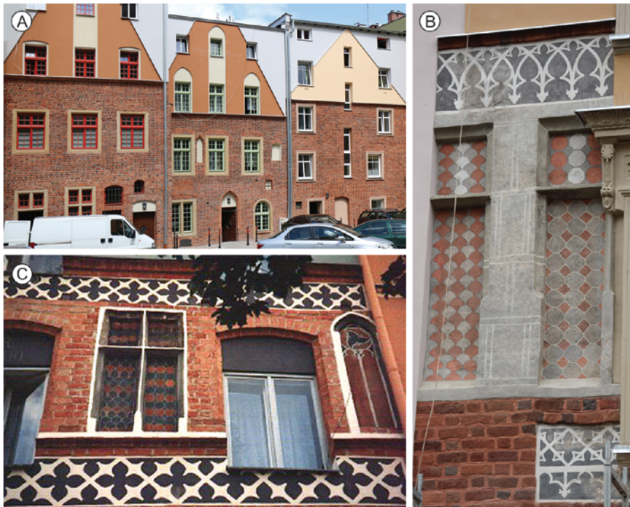
Fig. 79. Brzeg, elevations of tenement houses. A – 8–12 Dzierżonia Street, back elevation; B – 12 Dzierżonia Street, fragment of the facade on the first floor; C – 2 Rynek, facade on the first floor. Photo by M. Chorowska.
