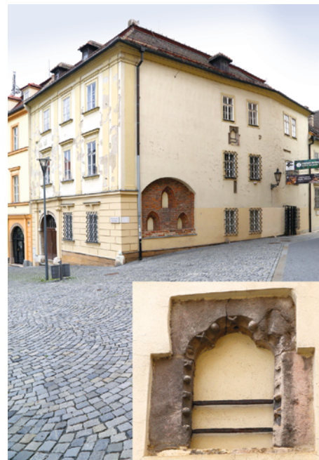
Fig. 109. Brno, 7 Zelný trh Square. Detail of early Gothic window on the second (?) floor. Photo by M. Peška.
