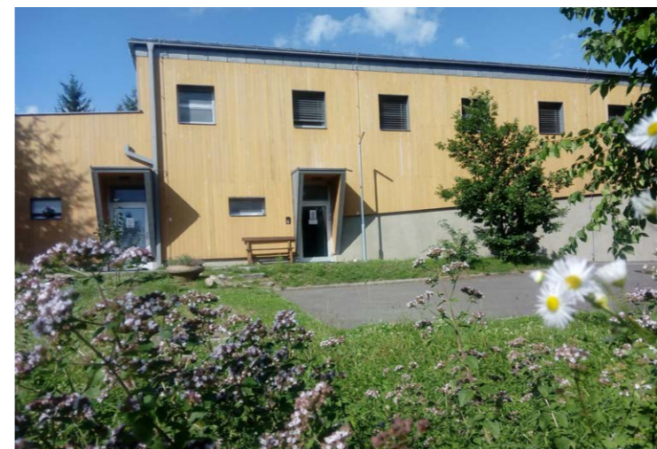
The mouse breeding facility in Studenec was fully reconstructed in 2017. | Photo from IVB archive
