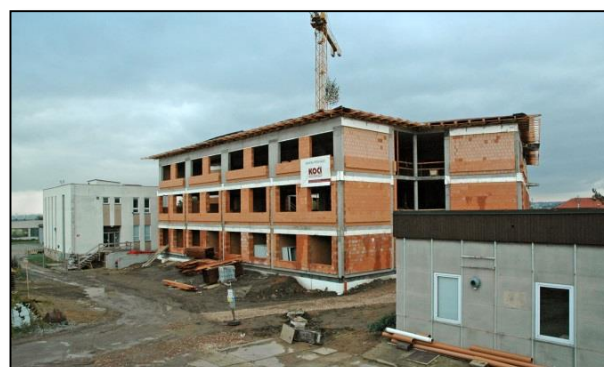
Construction of a new building.
