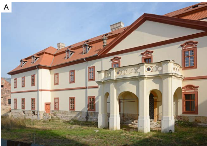
■ Fig. 30. Construction of the chateau at Konojedy (A) employed mostly dimensioned stone from the extensive sandstone quarries at Ústěček, as confirmed by the material study. In contrast, the later-built garden wall (B) was probably made of local material (Držovice Quarry). Photo by J. Adamovič.
