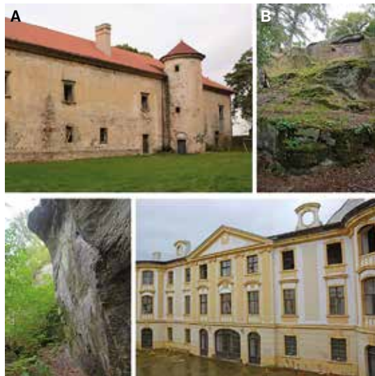
FIG. 42 Historical objects in the Zahrádky area and sandstone quarries producing the material for their construction. A – Vřísek, Renaissance chateau, B – Vřísek, a quarry at the N foot of the chateau, where dimension stone was taken, C – Nový Zámek, a quarry at the NW foot of the chateau, where dimension stone was extracted by undercutting and used for the Baroque rebuilding of the chateau, D – Nový Zámek, Renaissance chateau, recently damaged by fire. Photo by J. Adamovič.
